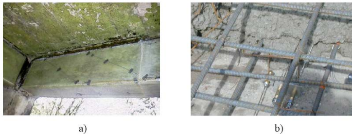
Fig 18 (a) Surface mounted fiber strain sensors on a bridge girder and, (b) sensor embedment into a concrete slab prior to curing.
